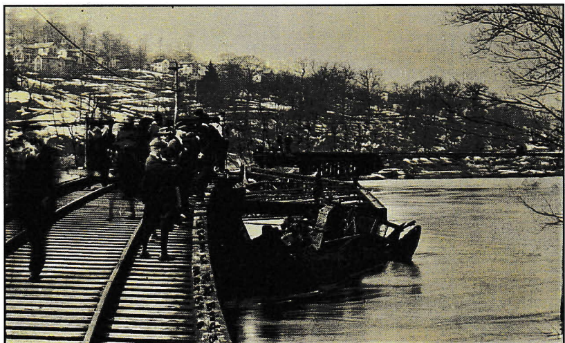
Meadville Evening Republican photo of B&LE #67 laying in French Creek after bridge collapsed. March 6, 1910
