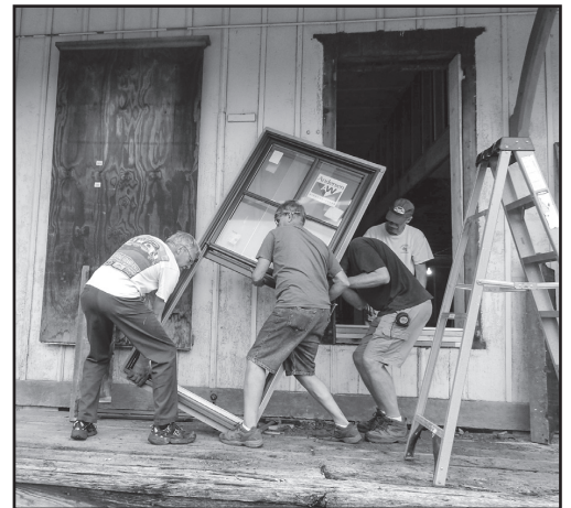
Crew hanging the first new window at the Meadville Railroad Depot. (Maryann Martin photo)
