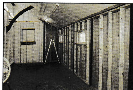
Former entrance room to be the kitchenette July 18, 2019 - © FCVRRHS
